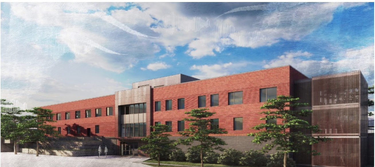
Foundry 2 Hub (Rushby Street)
